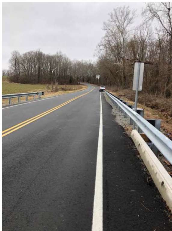
Looking West from Bridge
