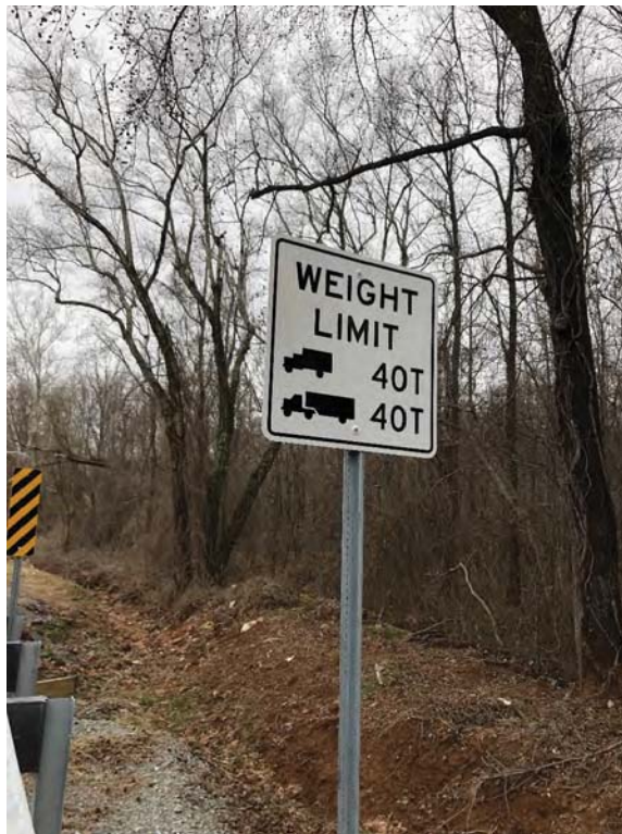
Weight Limit Sign at East Approach of Bridge
