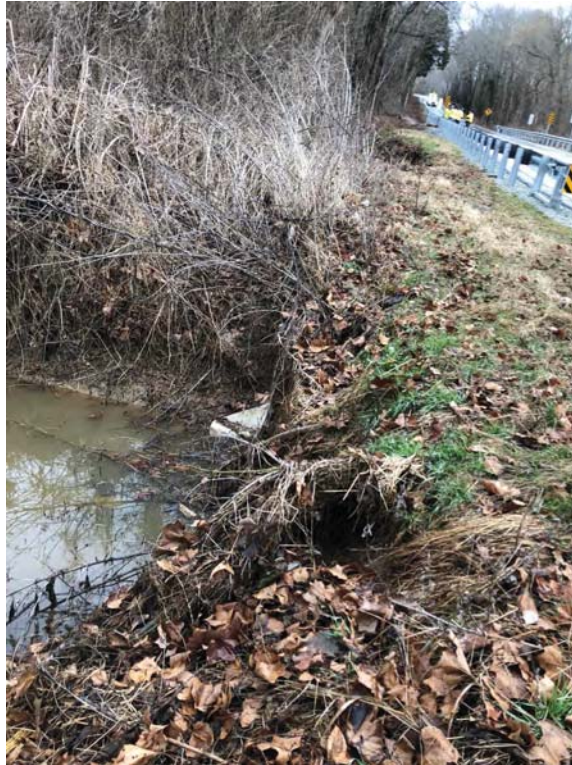
Flood Plain Downstream looking towards Bridge
