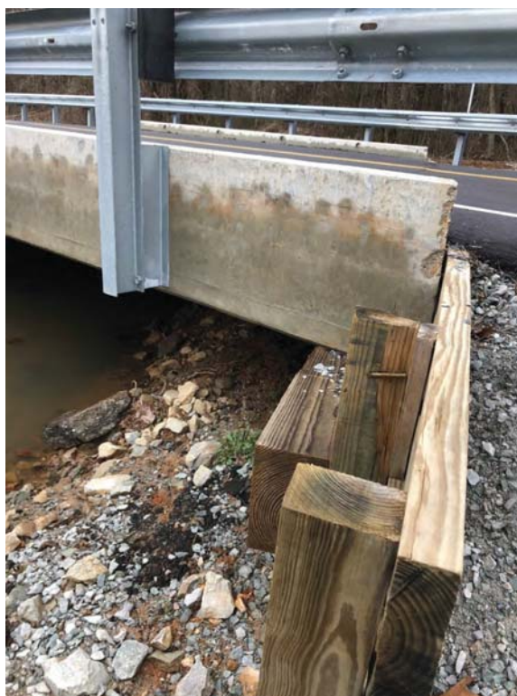
Connection to East Abutment on Inlet Side
