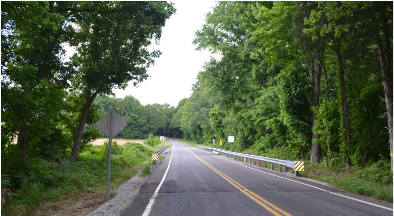
View west along SR-223 toward the bridge.
