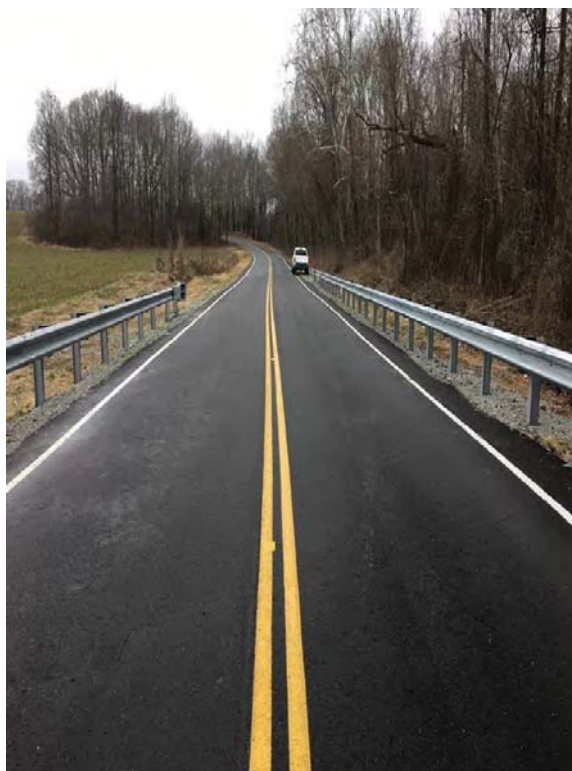
Westbound from Bridge
