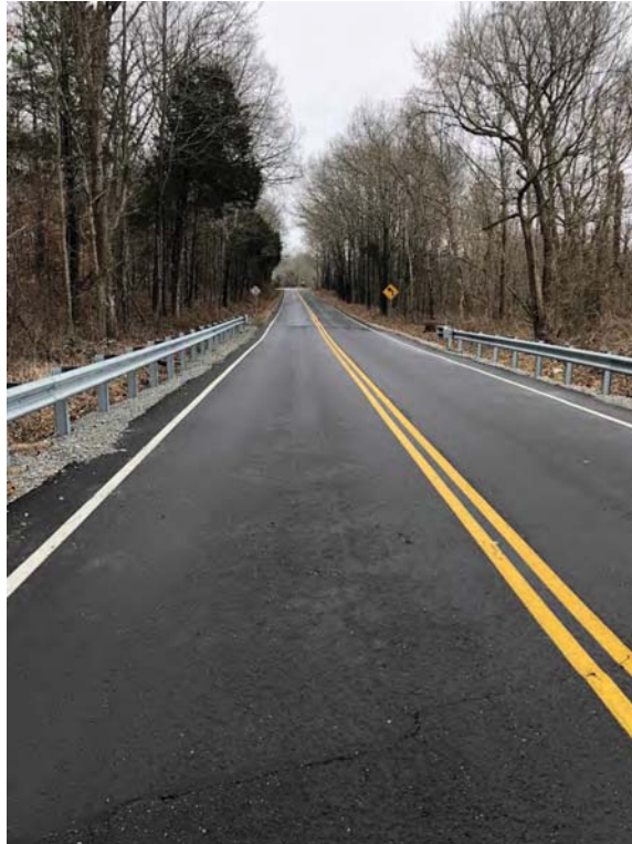
Looking East from Bridge
