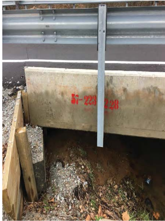
Connection to West Abutment on Inlet Side
