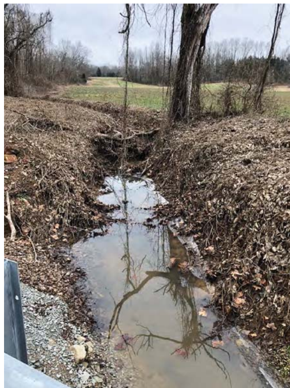
Upstream View from Bridge
